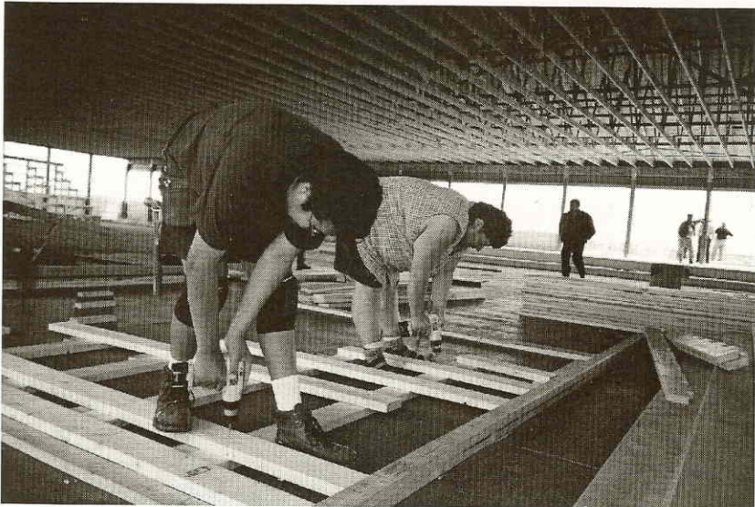
Students constructing bleachers at Batoche. GDI Archives (June 2001)
