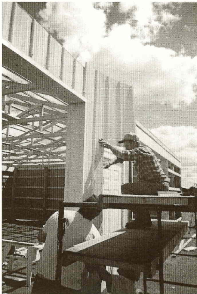
Elders Building Construction at Batoche DTI. 6DI Archives (June 2001)
